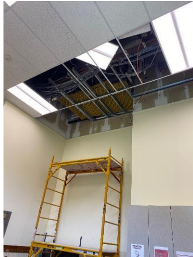
Tech room ceiling, during construction...
