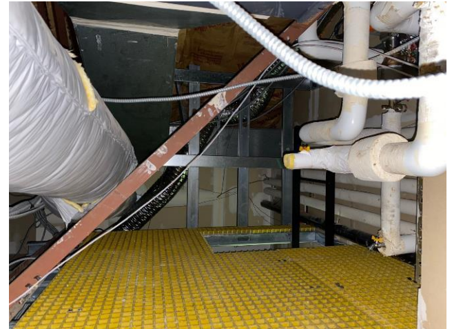
Ladder & platform, view from above the ceiling, after construction.
