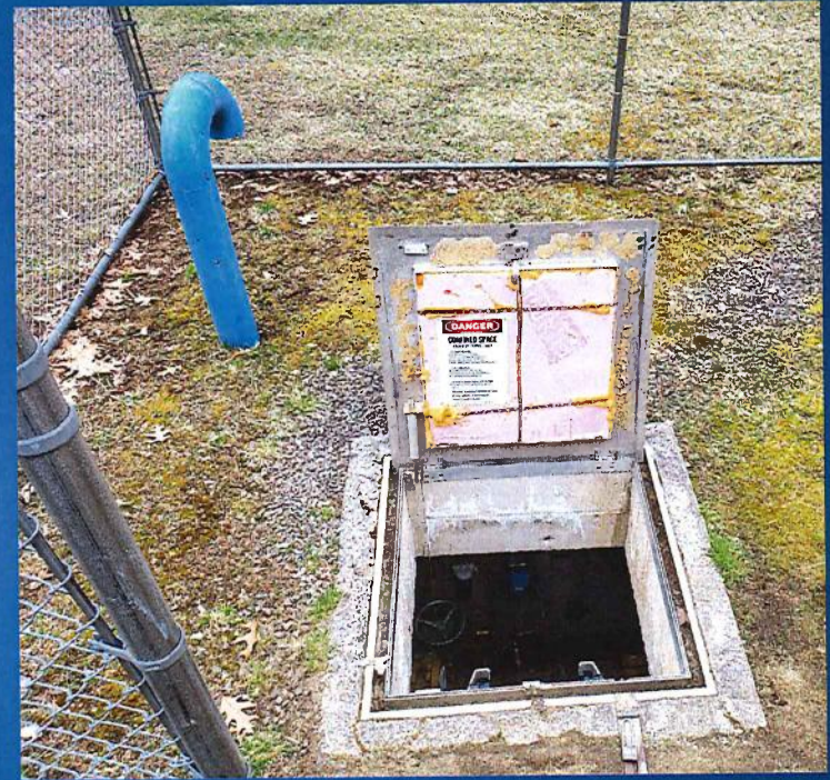
Image: Tank Vault
