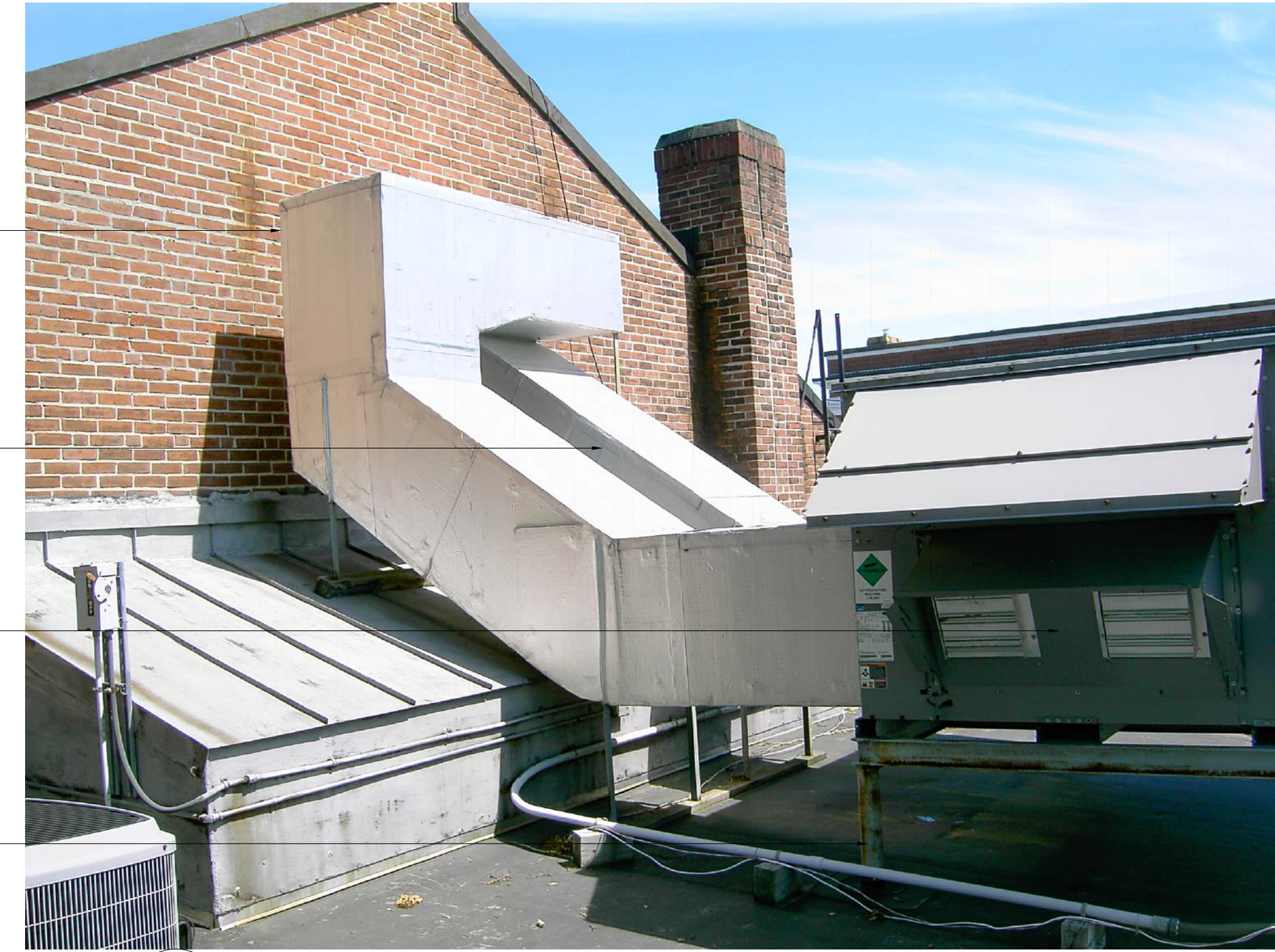
3 EXISTING RTU AND DUCT NOT TO SCALE
