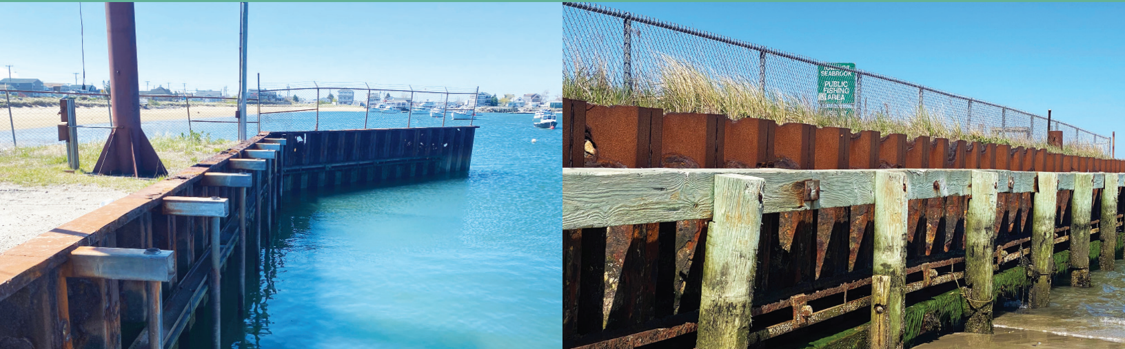
Seawall Project, Seabrook, NH.
