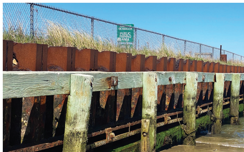
Seawall Project, Seabrook, NH.
