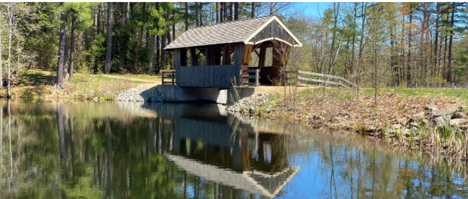
Pedestrian Recreation Bridge at Watson Pond, Chester, NH.
