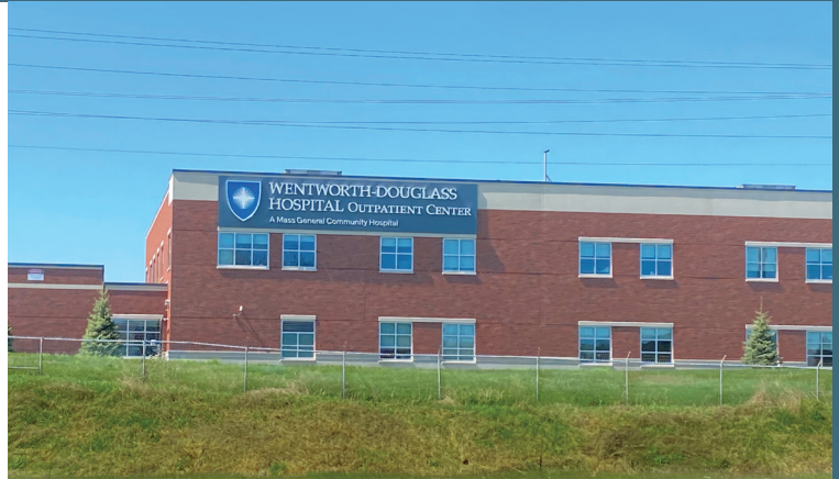
Wentworth-Douglas Hospital Portsmouth Outpatient Center, Portsmouth, NH.
