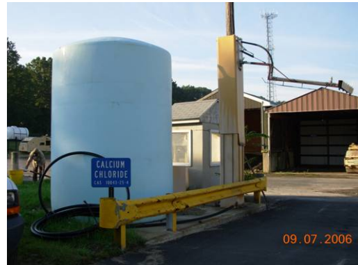
Figure 38. Overhead Pre-Wet Spray System
