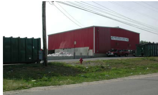
Derry Transfer Station, 40 Fordway
