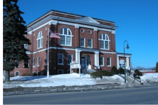
Adams Memorial Building, West Broadway
