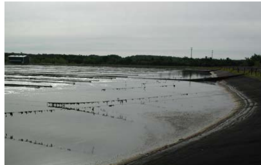
Wastewater Treatment Plant pond, Transfer Lane
