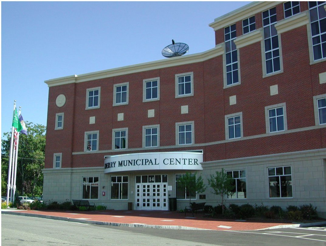
Derry Municipal Center and Emergency Management Center
