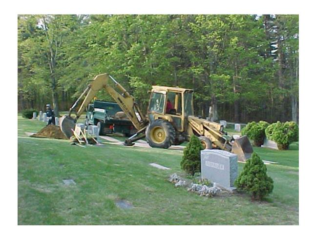
The backhoe is brought in across plywood so it does not create ruts on any of the existing plots. The equipment setup is a careful maneuver with the lack of space
