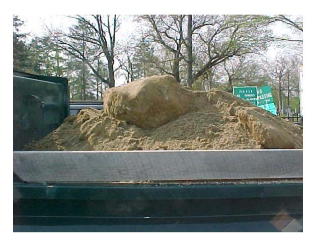
This dump truck bed has the fill removed from one gravesite. The photo shows large boulders and rock. With ledge, clay, and water we can only burry five feet deep. With rolling hills and a high water table, this makes winter burials very difficult. On some occasions,
