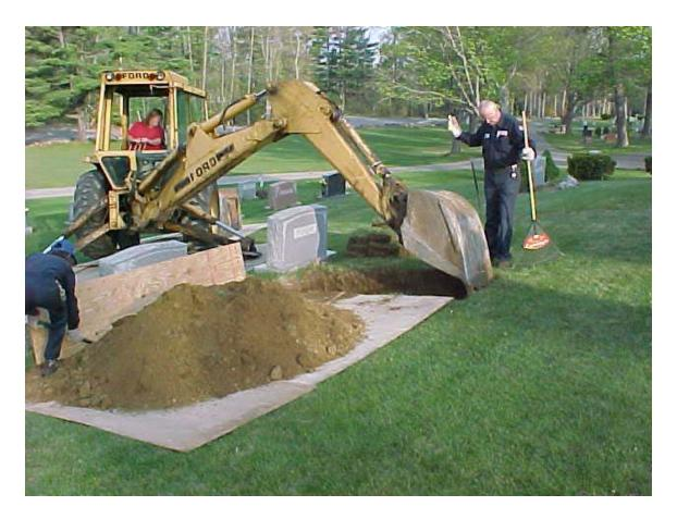
The staff acts as spotters for the backhoe. The dirt is saved and piled on to sheets of plywood. You can see the short distance between the monument and the hole.
